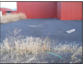
Asphalt Cap over soil contamination in Prineville
