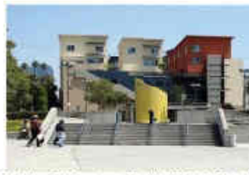
MacArthur Park Apartments, Westlake MacArthur Station, LA $16M TOD Loans, $3M TOD Grant 172 Affordable Units
