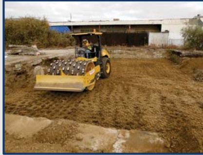
Compaction of backfilling Area 2
