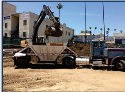
Loading backfill material
