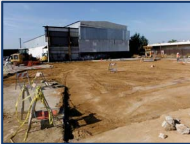
Backfilled prior to restoration of concrete paving
