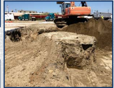
Excavation in Area 3
