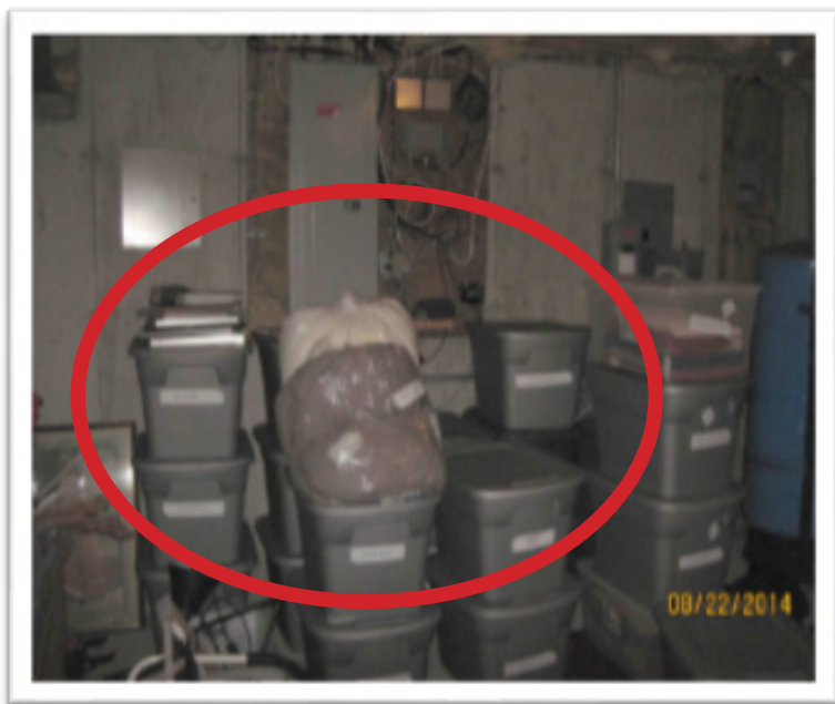
Photo D3: Working clearance not maintained: NEC 110.26
