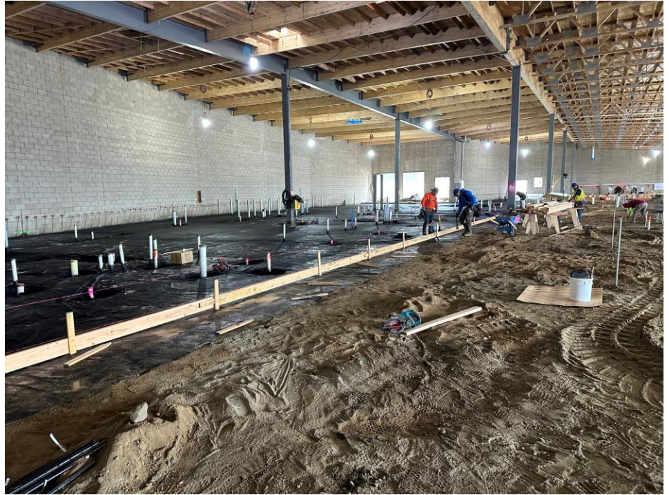
Installation of Vapor Barrier System – New construction
