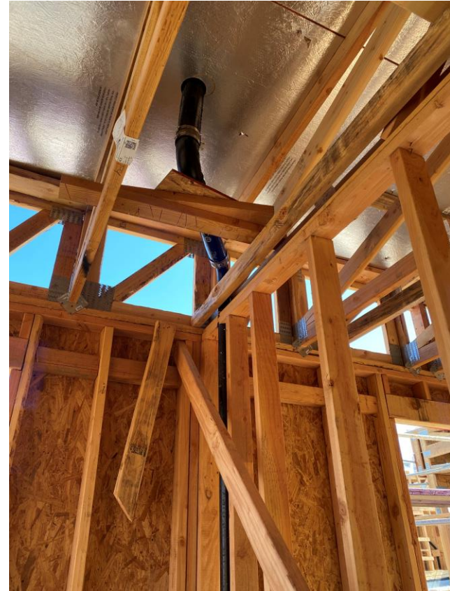
Vent riser of VIMS – residential construction
